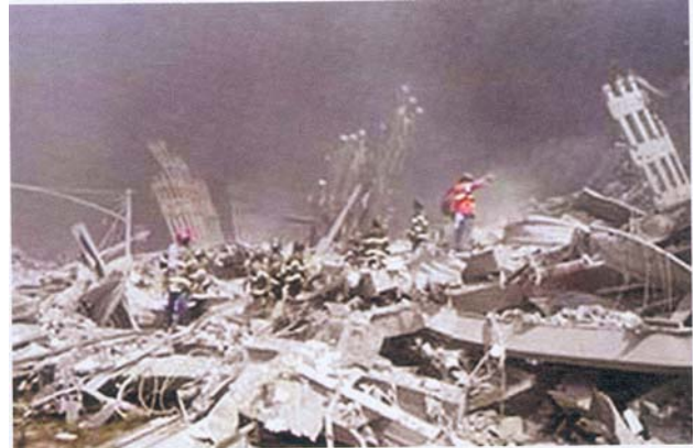
Figure 3. A representative photograph of the rubble pile at the epicenter of the collapse zone, also known as 'ground zero.' Note the hazards of sharp debris, open pits, active fires, and heavy smoke conditions.
